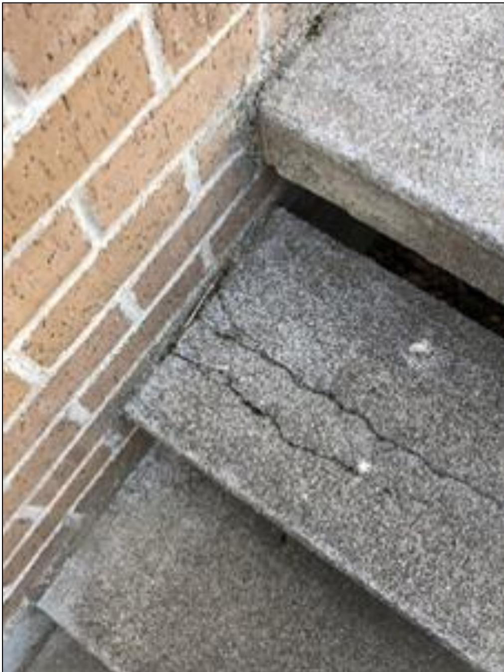
Figure 57. Fire Hall - Broken Stairs on North Door Landing
