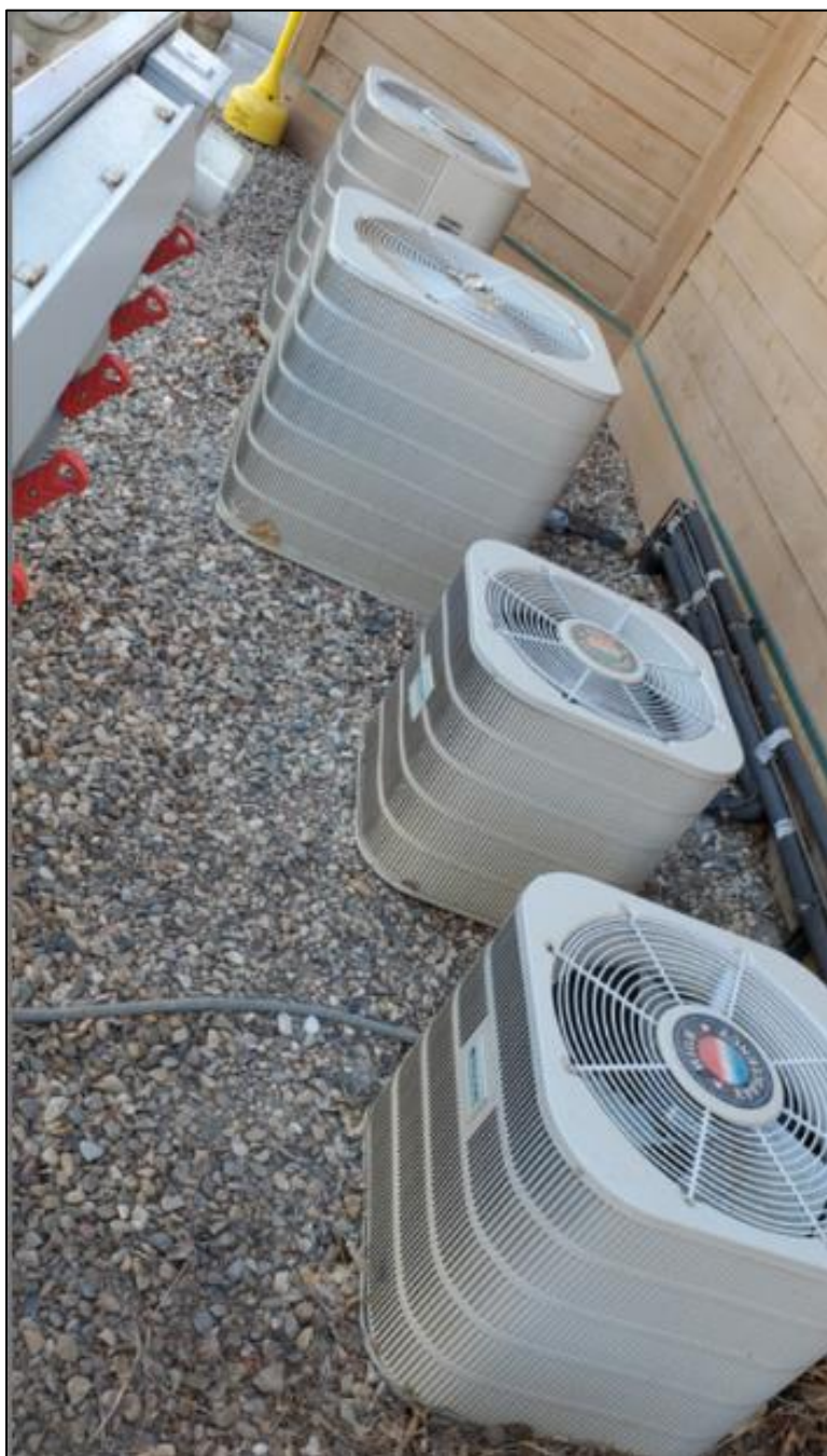
Figure 73. Visitor Center - Condensing Units
