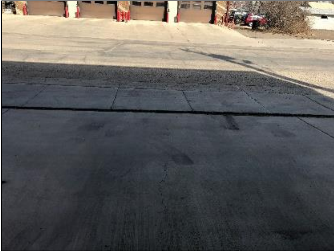
Figure 50. Emergency Services Building - Heaving Sidewalk in Building Front
