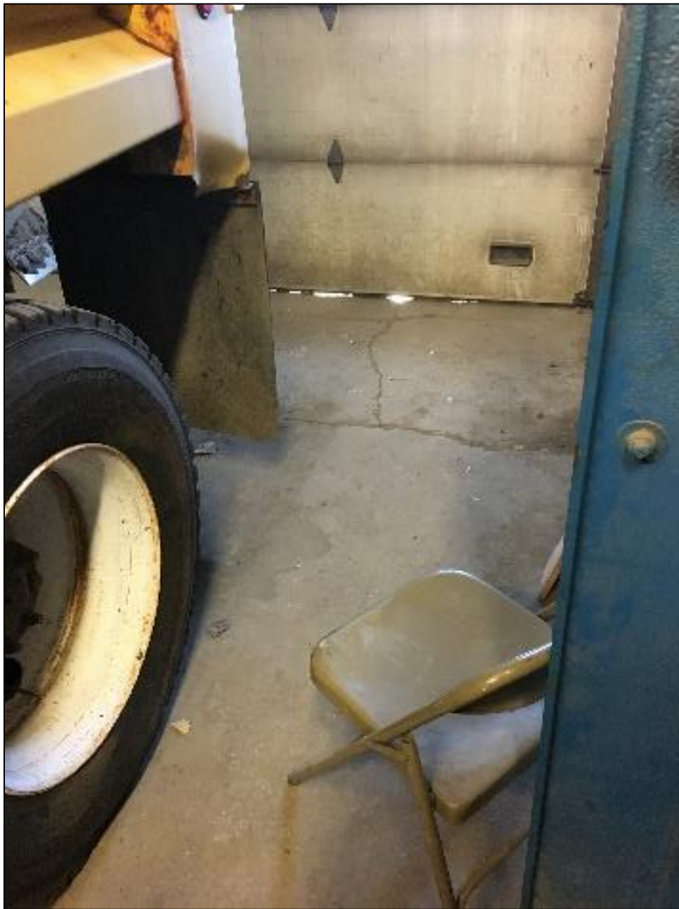
Figure 44. City Shops (Old) - Large Gaps Under Aging Garage Doors
