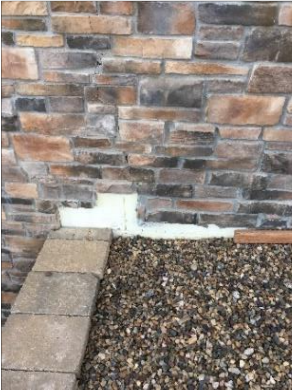
Figure 59. Fox Hills Clubhouse - Exposed Insulation Due to Missing Cultured Stone
