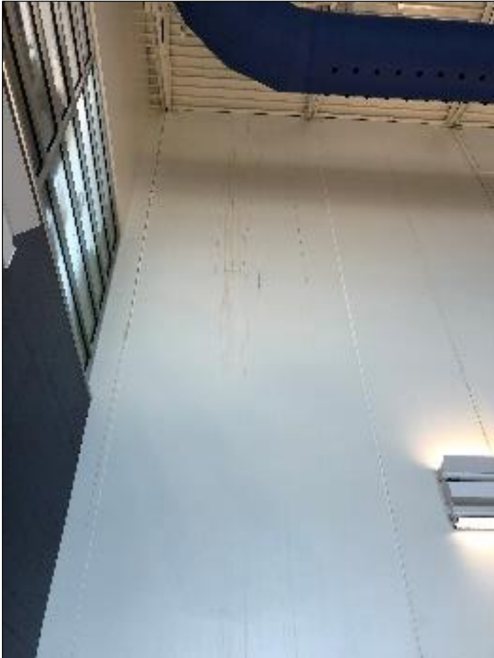
Figure 65. Rough Rider Center - Staining on Precast Walls
