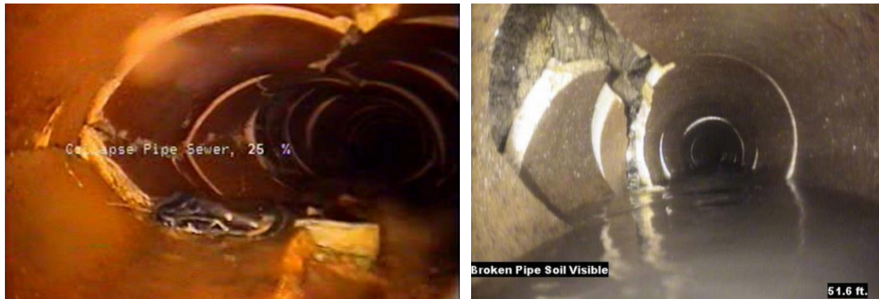
Figure 32. VCP Defect Examples (Left – Collapsed Sewer ; Right – Broken Pipe Soil Visible)
