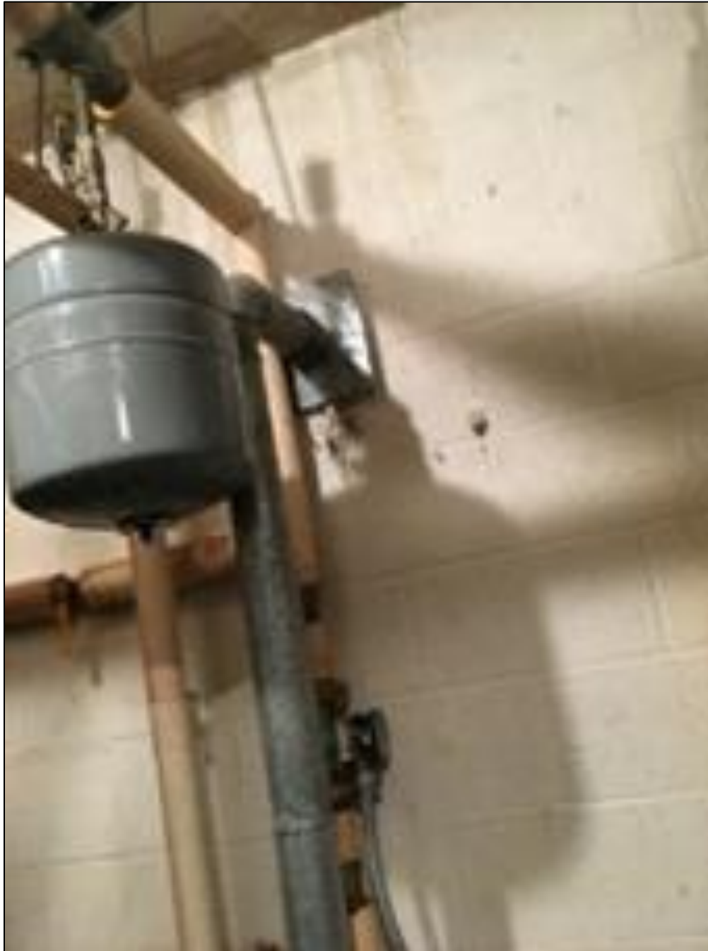
Figure 53. Fire Hall - Gap Between Mechanical Pipe and Exterior Wall
