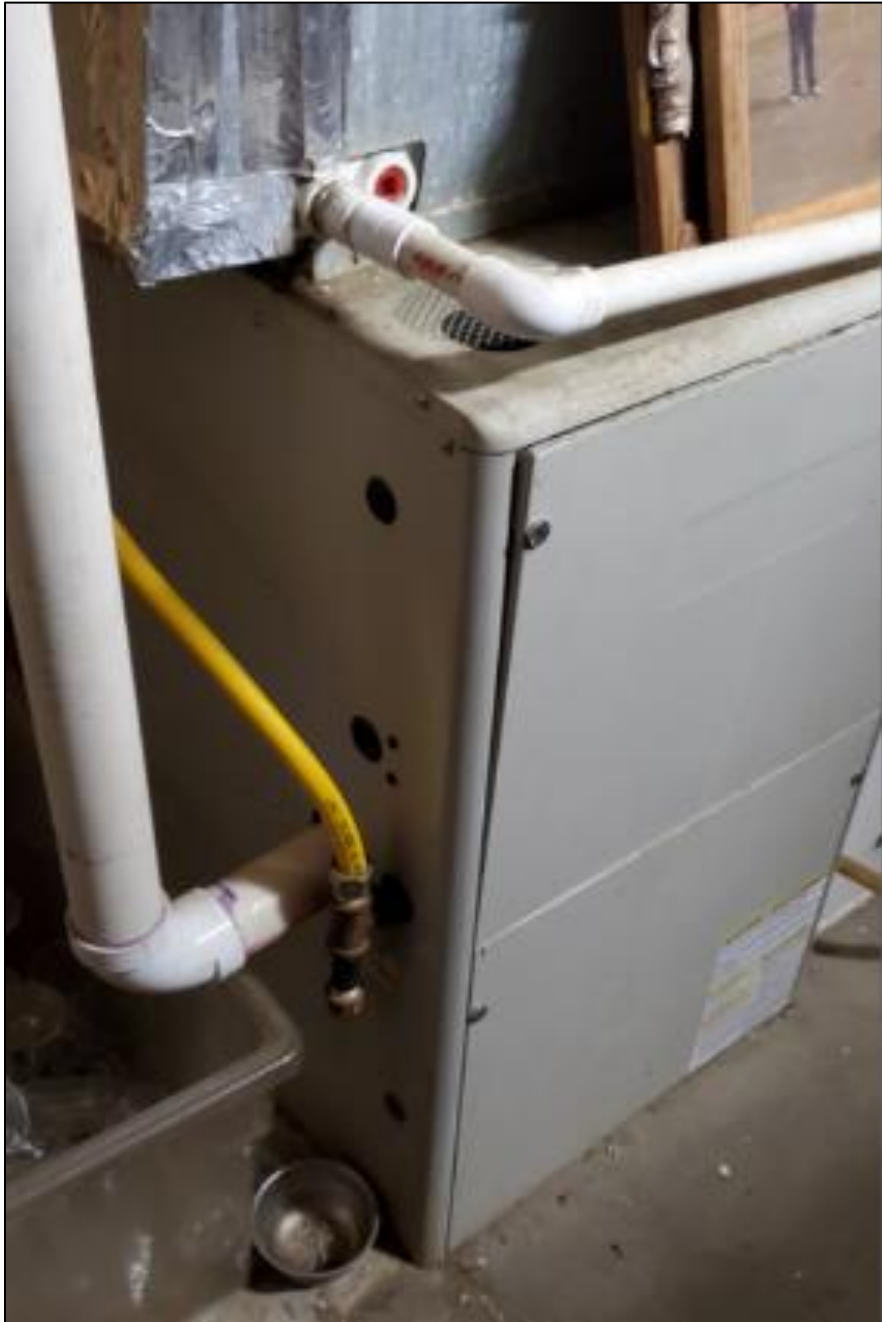
Figure 63. Fox Hills Clubhouse - Aging Gas-Fired Furnace
