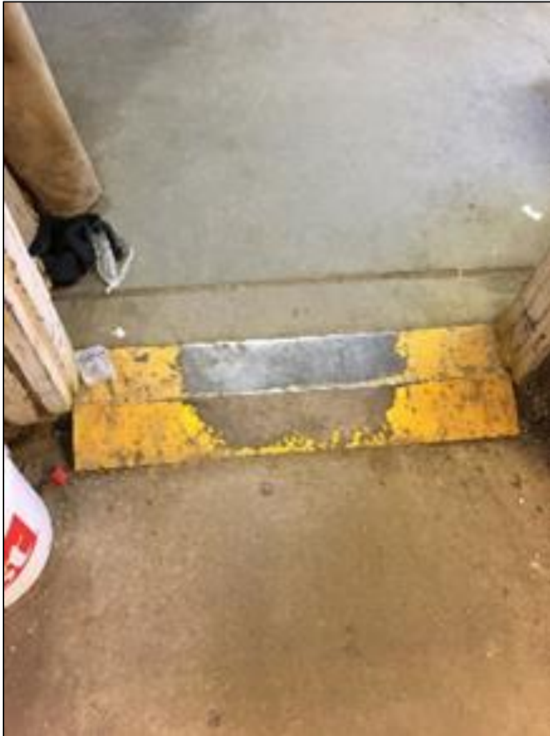
Figure 46. City Shops (Old) - Interior Step Showing Signs of Wear
