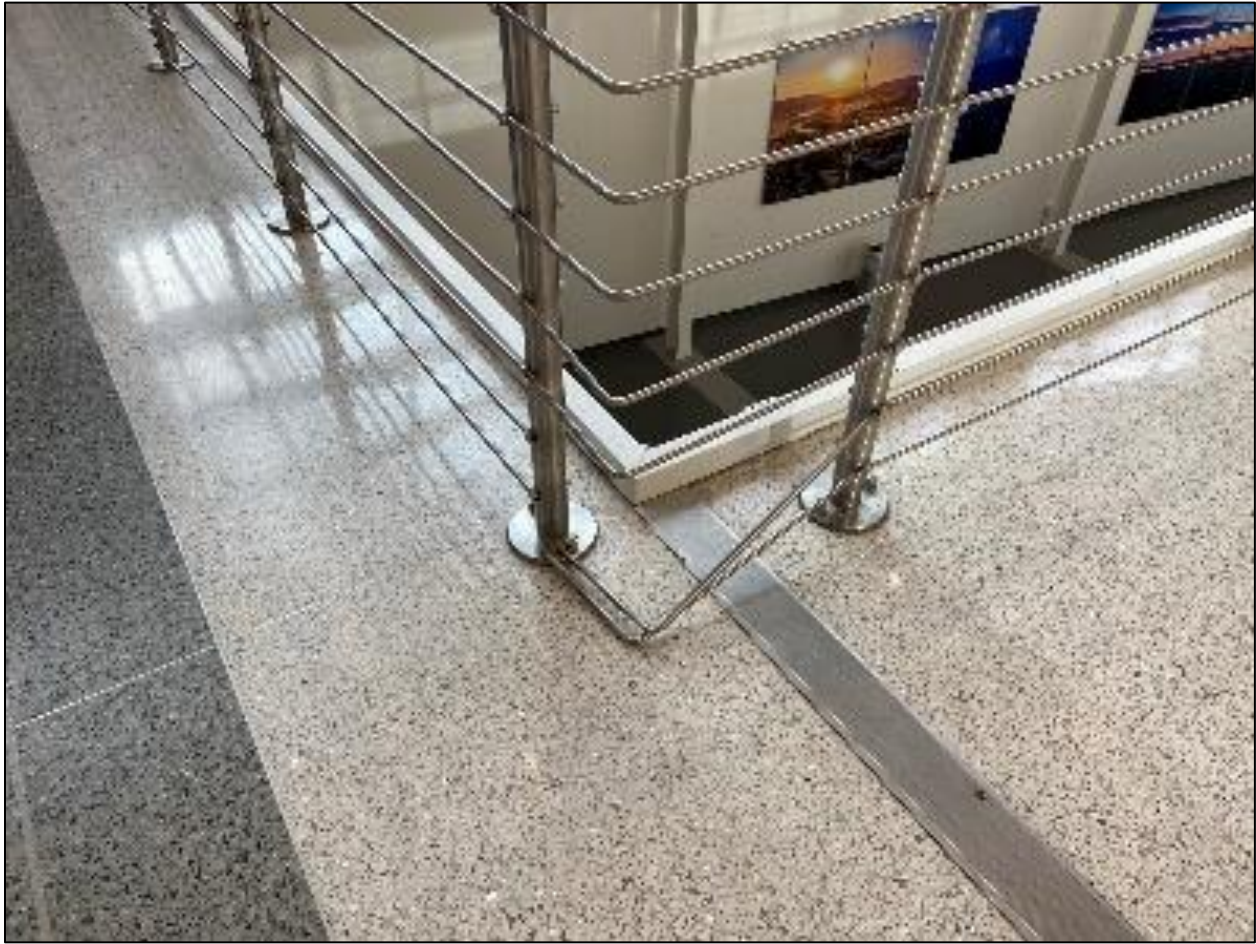
Figure 67. Rough Rider Center - Broken Horizontal Rails on Rough Rider Center Railings
