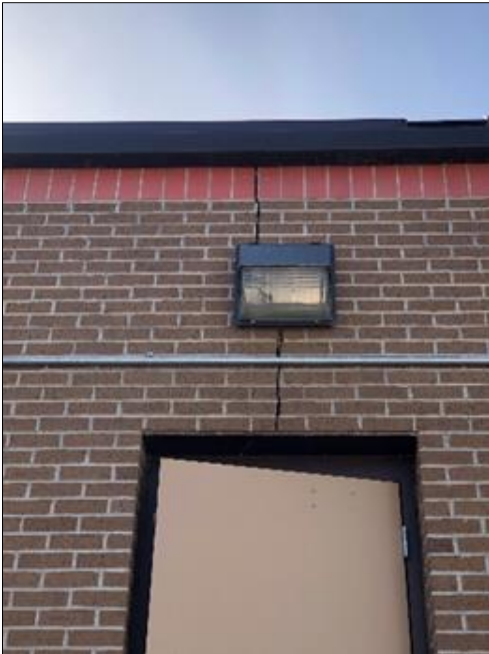
Figure 52. Fire Hall - Crack Above North Door
