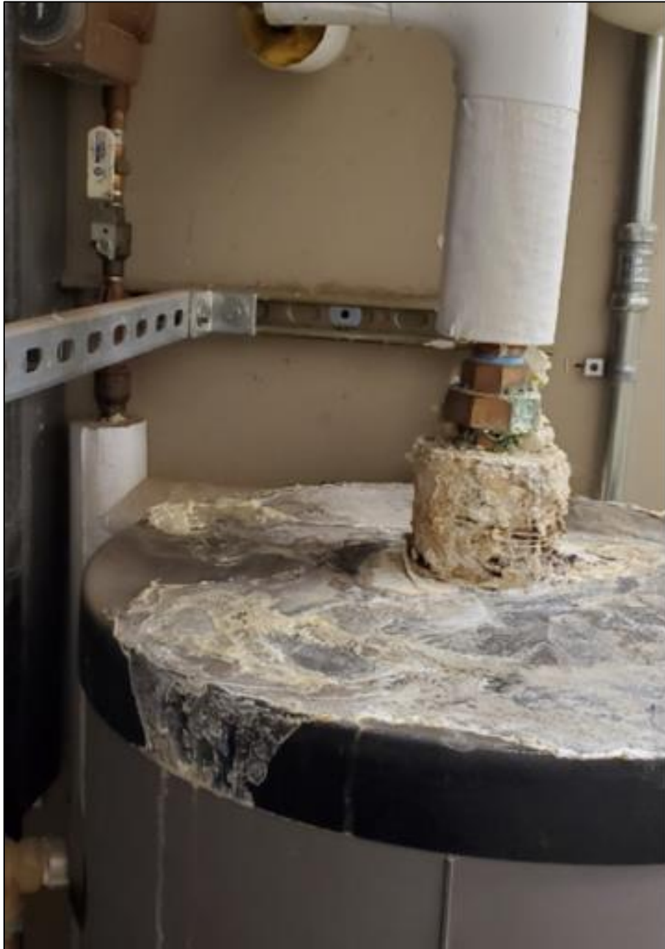
Figure 51. Emergency Services Building - Sediment Buildup on Water Heater
