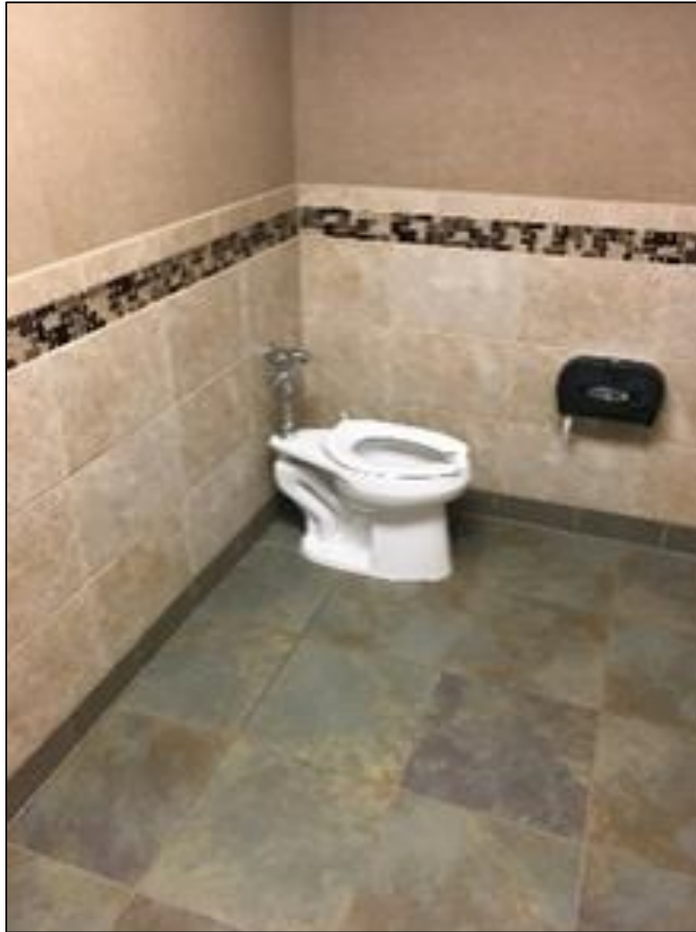
Figure 42. City Hall and Civic Center - Lower Restroom Missing ADA Grab Bars
