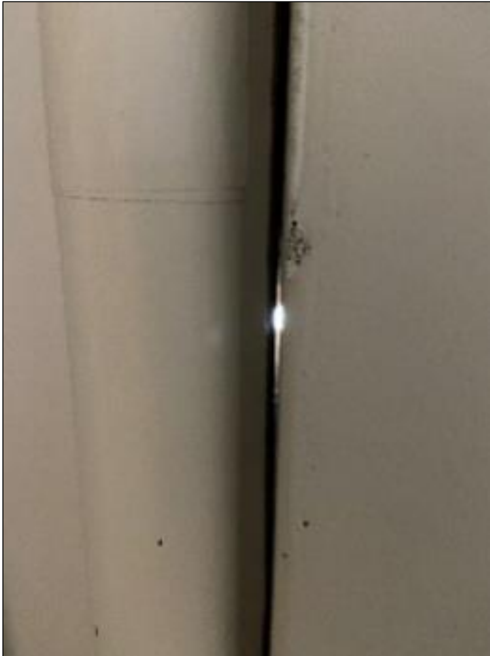
Figure 64. Rough Rider Center - Gap Between Precast Panels in Hockey Arena
