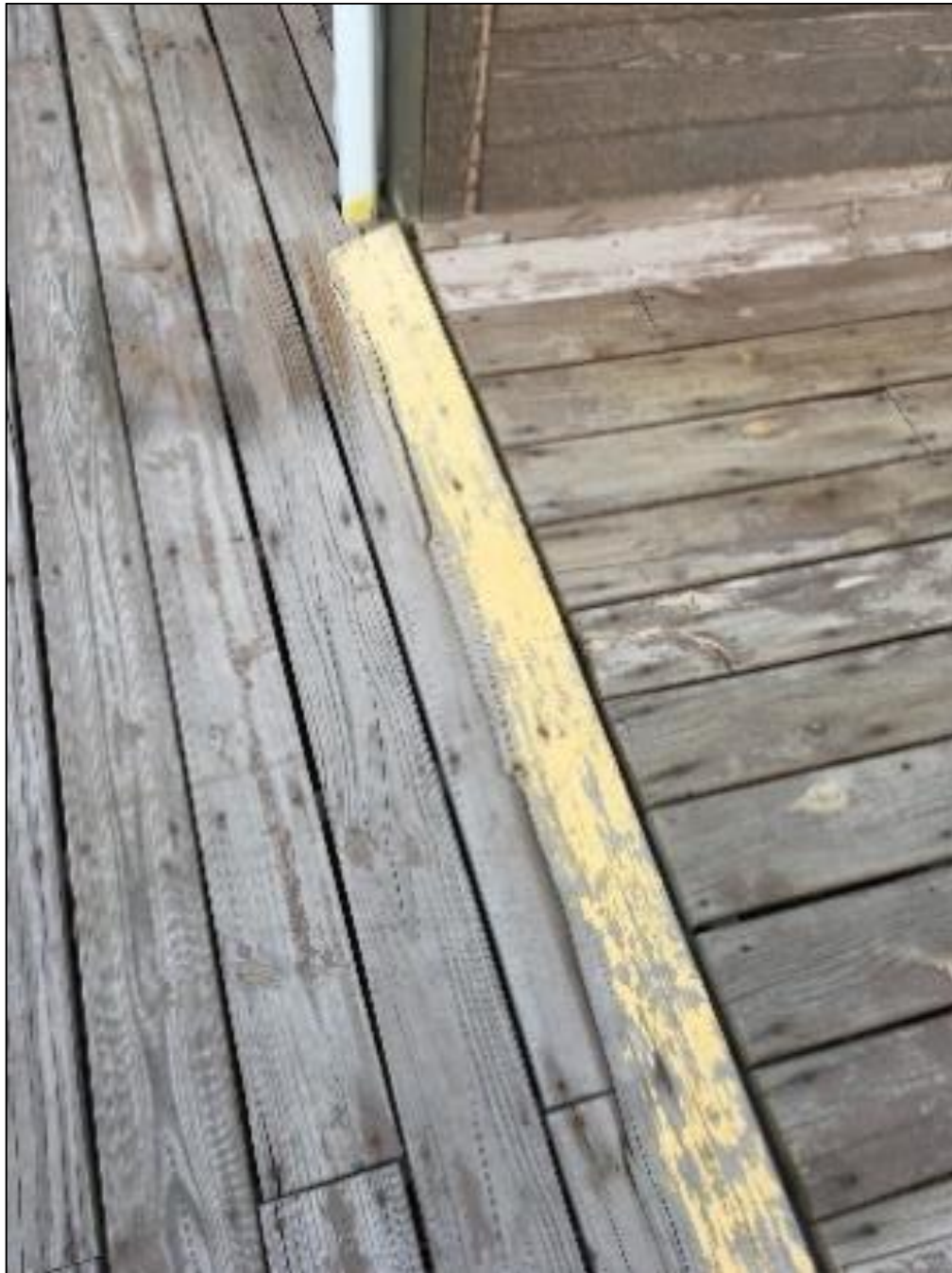
Figure 61. Fox Hills Clubhouse - Elevation Difference Between South and East Deck
