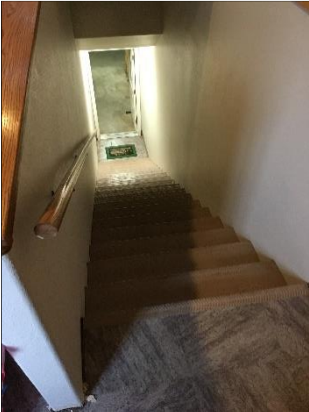
Figure 60. Fox Hills Clubhouse - Missing Handrail on Basement Stairs
